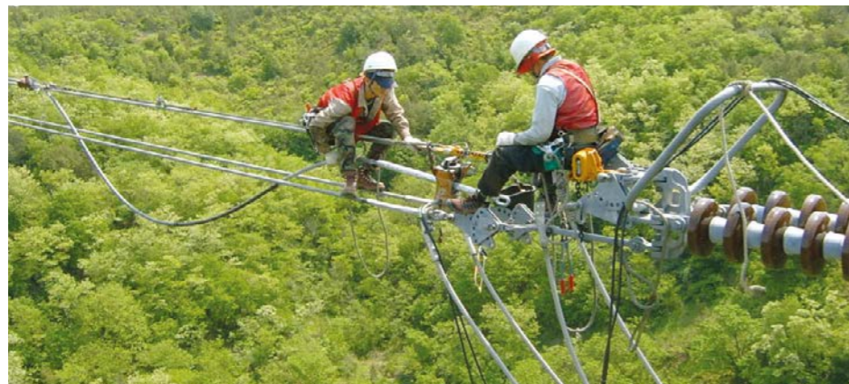
765kV Insulator String Set & Fittings
